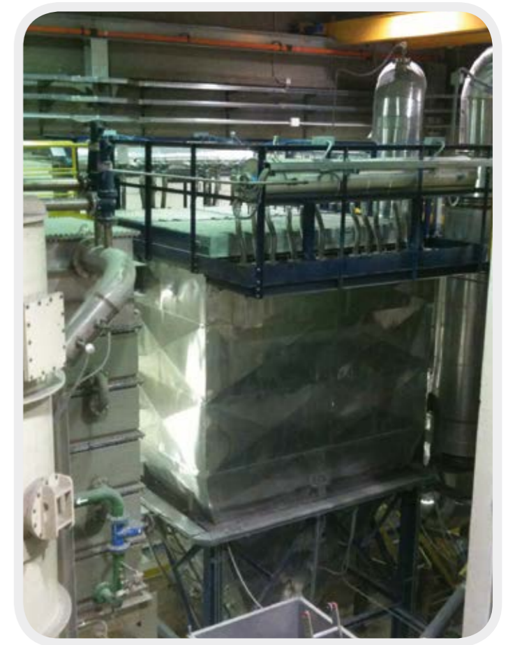
Particulate matter filter
